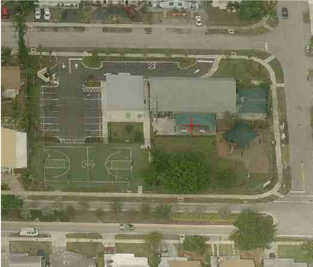
NORTH ANDREWS GARDENS COMMUNITY CENTER 250 NE 56TH CT
