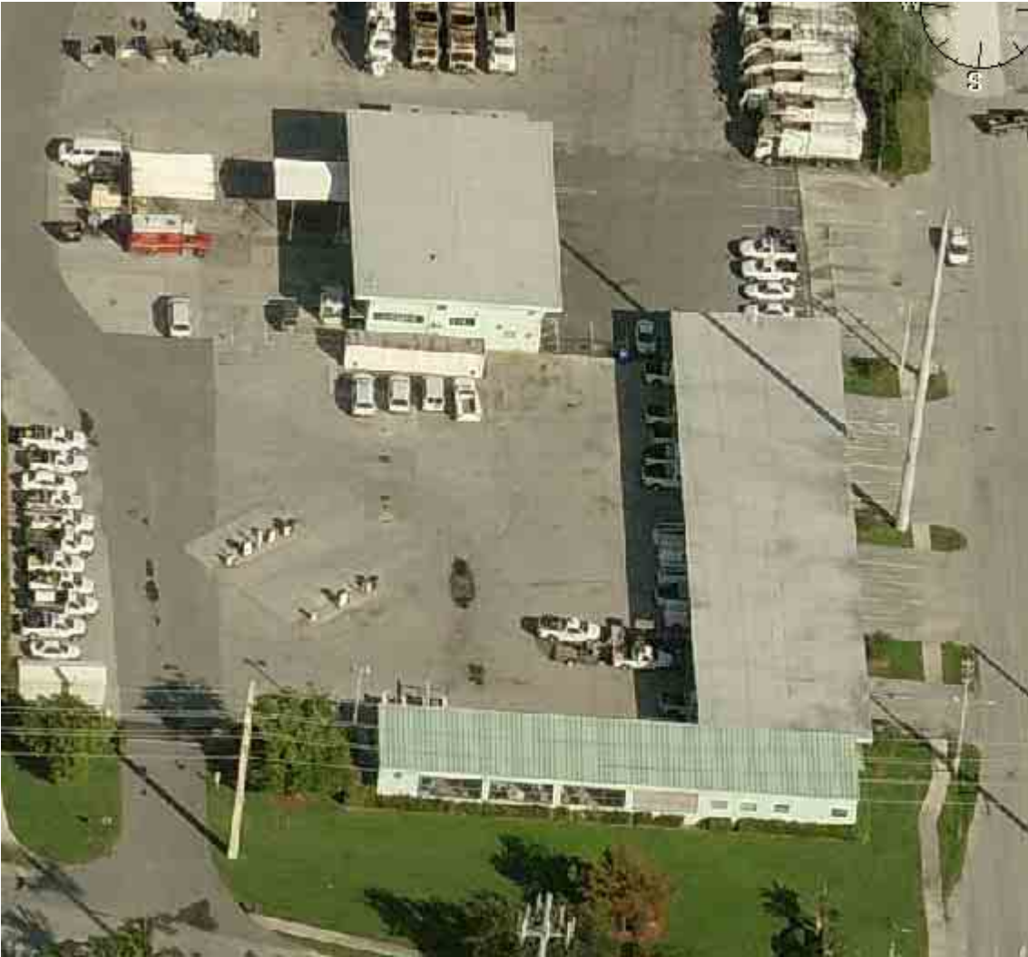
MUNICIPAL SERVICES BUILDING and GARAGE 3801 NE 5TH AV
