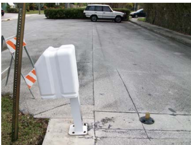
Old Gate arm structure damaged
